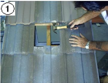
**2A. Straight bonded roof:-** Knock tile lugs off bottom of tile in the course above to allow the tile to sit flush with the vent.
