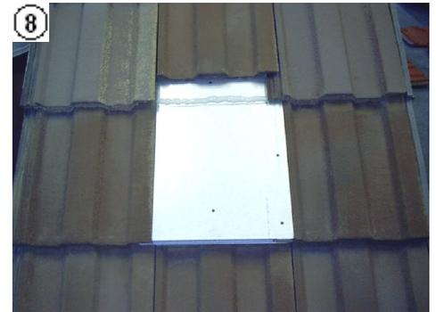
9. Pull the tile/s back into position, smooth the silicon out to close all gaps between vent and tile/s (**Be careful not to block out any water courses**). Finally, run a bead of silicon down both sides of the vent attaching the tiles to the vent. The water courses above vent may also be silicon sealed if preferred.
