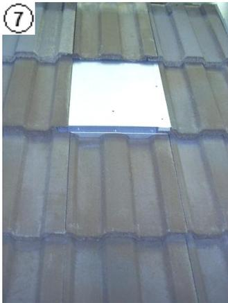
7. Install the vent in place making sure that the trimmed out flap fixes under the right hand host tile.
